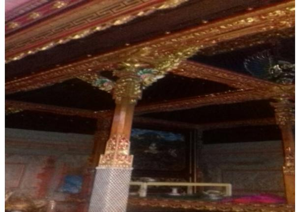
**Gambar 6.** Detail Konstruksi Bale Delod (Sakutus) bertiang 8
